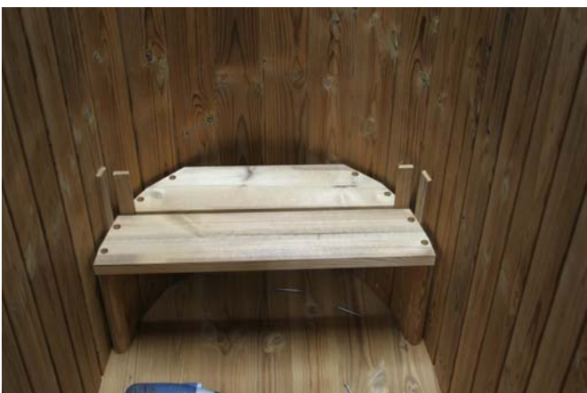
Continue with the next seat, use the "calibration pieces" as shown in the picture and repeat the previous steps.
