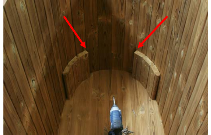
Place the first support piece at the third stave, as the arrow indicates. See picture on the last page for more details. Screw all pieces into the walls.
