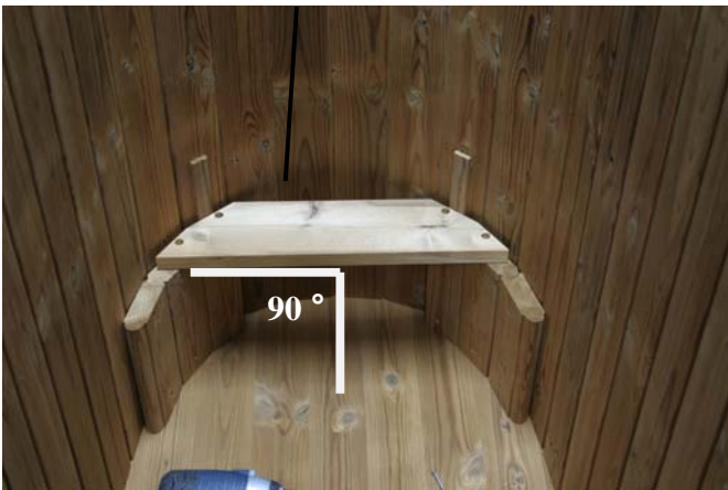
Place the first seat, the included "calibration pieces" help to align the seat properly. Check that the seat is at a 90 degree angle with the bottom.
