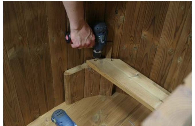
Predrill with 3mm drill and then attach the seat with 4 screws, don't forget to use the included washers!
