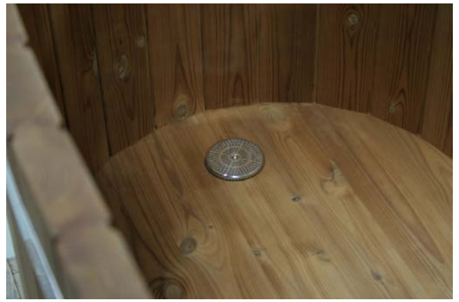
Finally attach the grill for the drainage hole.
