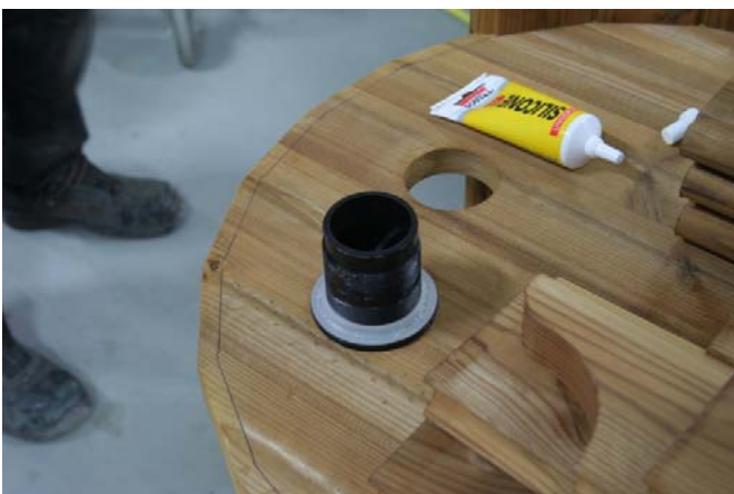
Smear out the silicone on the threads with a finger.
