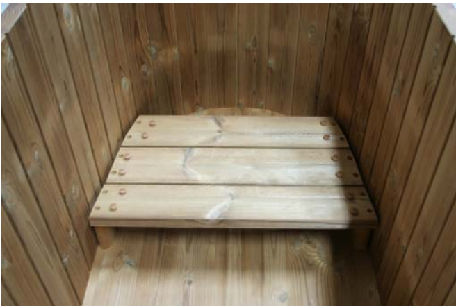
After all the benches are assembled, plug the hole with the included plastic plugs.
