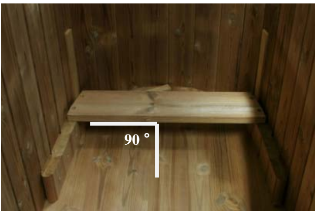
Now place the first bench. The included "calibration pieces" help align the bench correctly. Check that the bench is at a 90° angle with the base.
