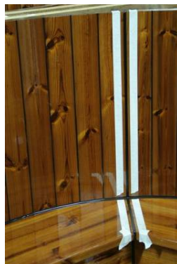
5. When the side modules are assembled and the sealing mass has dried for at least 6 hours, the vertical joints and the joint between the seat and side should be coated using the method illustrated earlier. Let it dry for at least 12 hours before checking for leakage. If the application of coating is made after the bath has been in use then the coating should be applied only after the joints, and a small area out from this, are cleaned with acetone and sanded.
