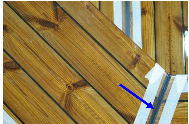
3.1 Lightly sand inside the masking
