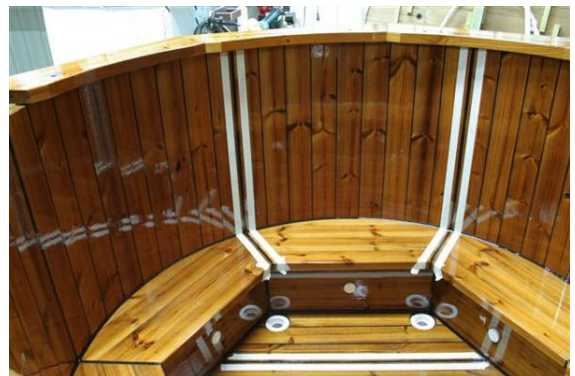
5. When the side modules are assembled and the sealing mass has dried for at least 6 hours, the vertical joints and the joint between the seat and side should be coated using the method illustrated earlier. Let it dry for at least 12 hours before checking for leakage. If the application of coating is made after the bath has been in use then the coating should be applied only after the joints, and a small area out from this, are cleaned with acetone and sanded.
